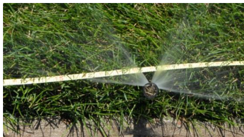
Verify spacing between heads with a tape measure. At 30 psi spray heads should be spaced at no greater than their series, i.e 15 series at 15 ft, 12 series at 12 ft, etc.
