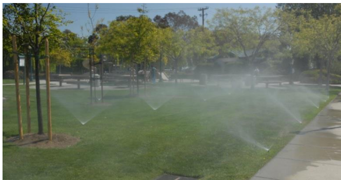
Spray heads operating at 90 psi. This problem was corrected with the addition of a regulator feature on the valve.
