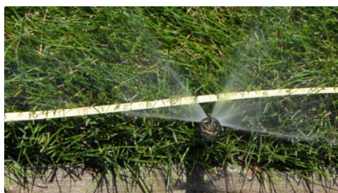
Verify spacing between heads with a tape measure. At 30 psi spray heads should be spaced at no greater than their series, i.e 15 series at 15 ft, 12 series at 12 ft, etc.
